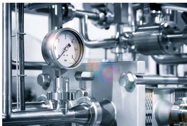
Figure 3. Pressure gauges are an invaluable and inexpensive tool for monitoring the performance of the system. Take care to protect the gauges by installing sufficient tubing to dissipate heat.
