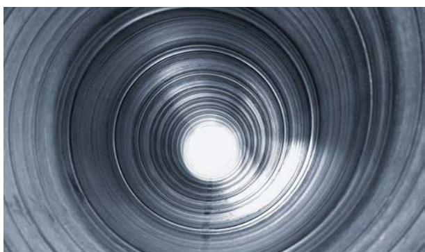
Figure 2. Multi-pass helical coil fired heaters are widely used in heat transfer applications for their thermal efficiency. Ensure that the maximum temperature ratings on the fluid are capable of handling the radiant heat generated inside the firebox for all fired heater designs.
