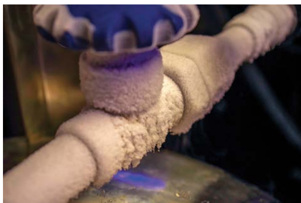
Figure 1. When selecting an appropriate heat transfer fluid, the ambient environment of the system must be accounted for. If any of the system is located outdoors, low temperature startup conditions may apply.
